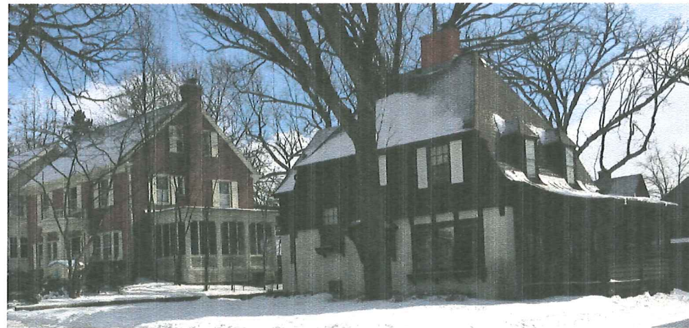
ADJACENT HOMES WITH WOOD FRAMED PORCHES
