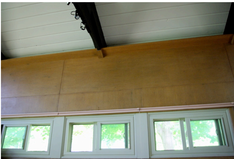
1954 U-Form-It by Erdman, Flambeau Rd. Interior windows, wall, ceiling detail.
