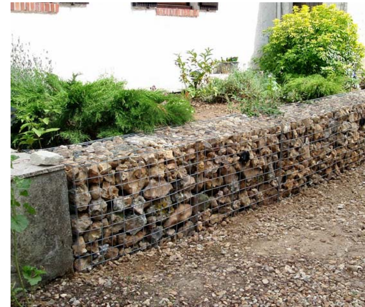
GABIAON ACCENT WALLS
