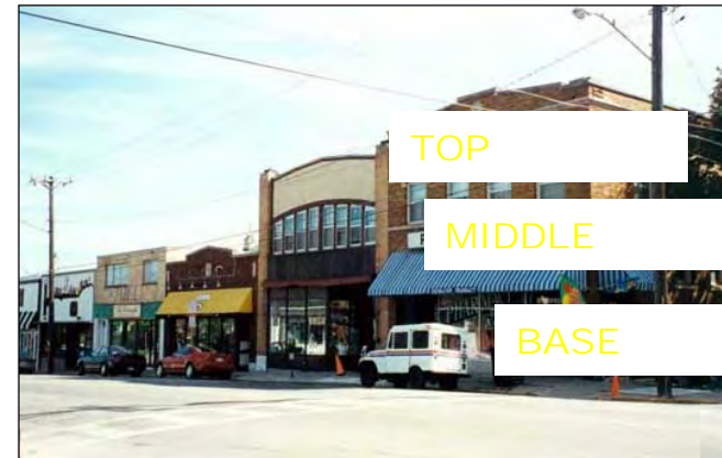
Figure J-2: Expression of Base, Middle, and Top in Existing Monroe Street Buildings
