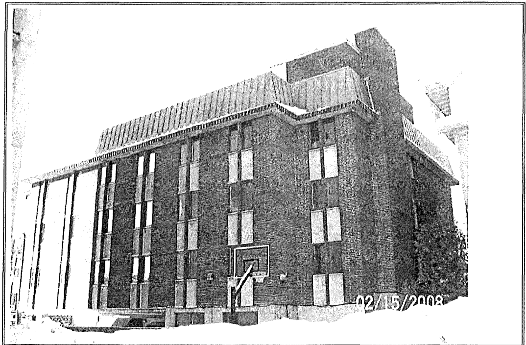
Photograph Number 4: East side elevation where chimney is located, note penthouse at roof.
