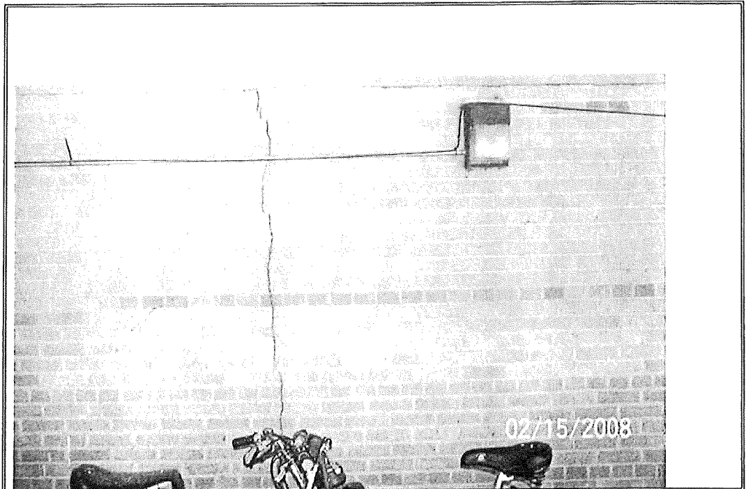
Photograph Number 16: Vertical masonry veneer cracks at east wall of carport.
