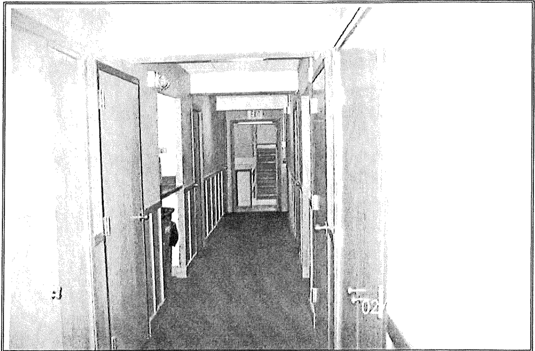
Photograph Number 29: Typical second and / or third floor hallway conditions.
