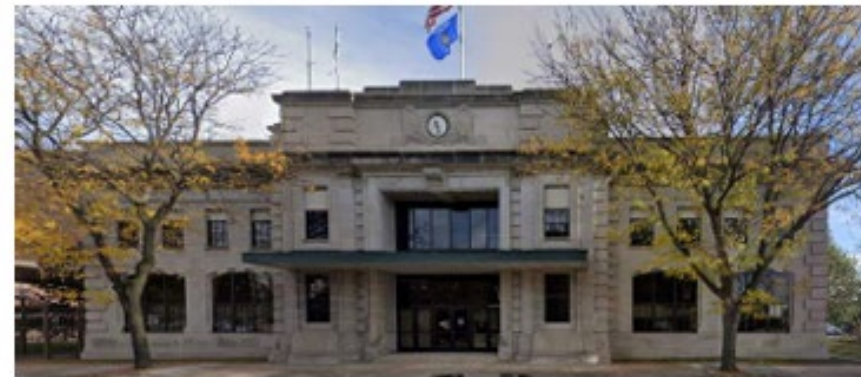
631 RAILROAD ST. FLAT ROOF, MASONRY, DOUBLE-HEIGHT ENTRY EXPRESSION, BASE WAINSCOT, CORNICE EXPRESSION, WINDOW GROUPINGS, RELATIVE SCALE, BEAUX ARTS STYLE, ARCHED WINDOWS
