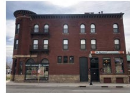
524 E. WILSON ST. FLAT ROOF, MASONRY, BASE WAINSCOT, WINDOW PROPORTIONS, RELATIVE SCALE, ARCHED WINDOWS
