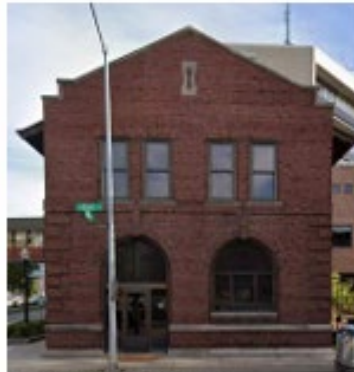
631 RAILROAD ST. MASONRY, BASE WAINSCOT, WINDOW GROUPINGS, ARCHED WINDOWS
