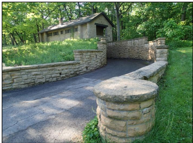
During the Great Depression, the Works Progress Administration and Civil Works Administration built stone entrances, the shelter, and fireplaces at Hoyt Park.
