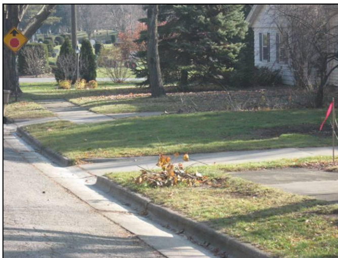
Missing sidewalk segments should be installed to improve safe pedestrian movement.
