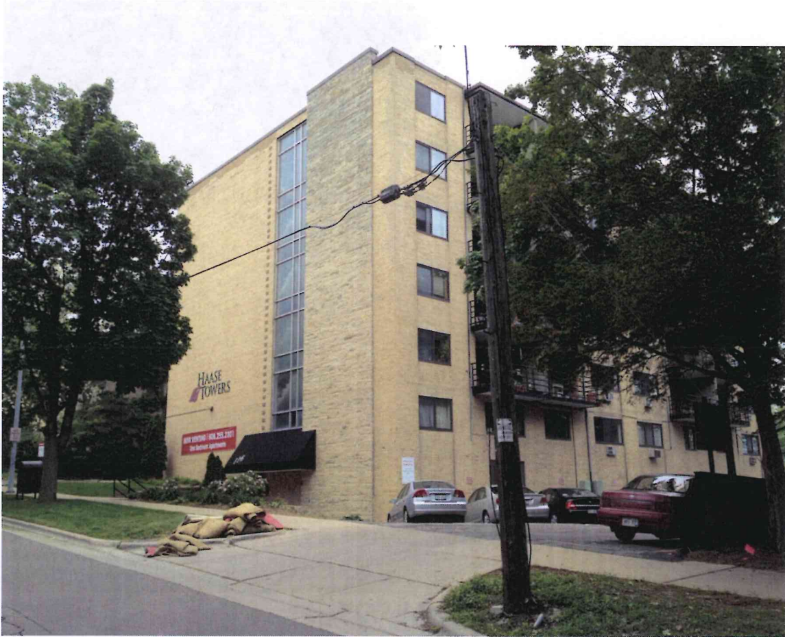
Residential apartment building to the south
