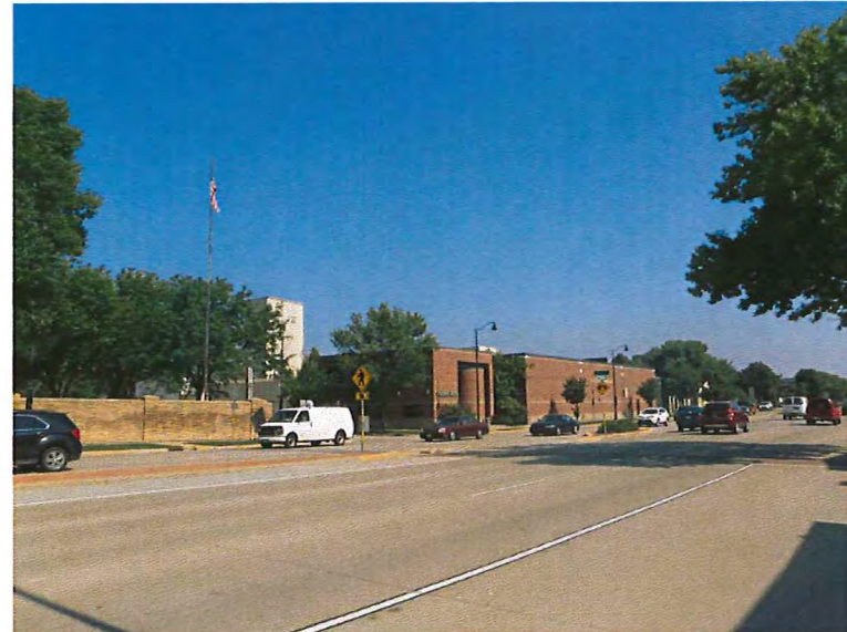
VIEW FROM EAST WASHINGTON LOOKING NORTHEAST
