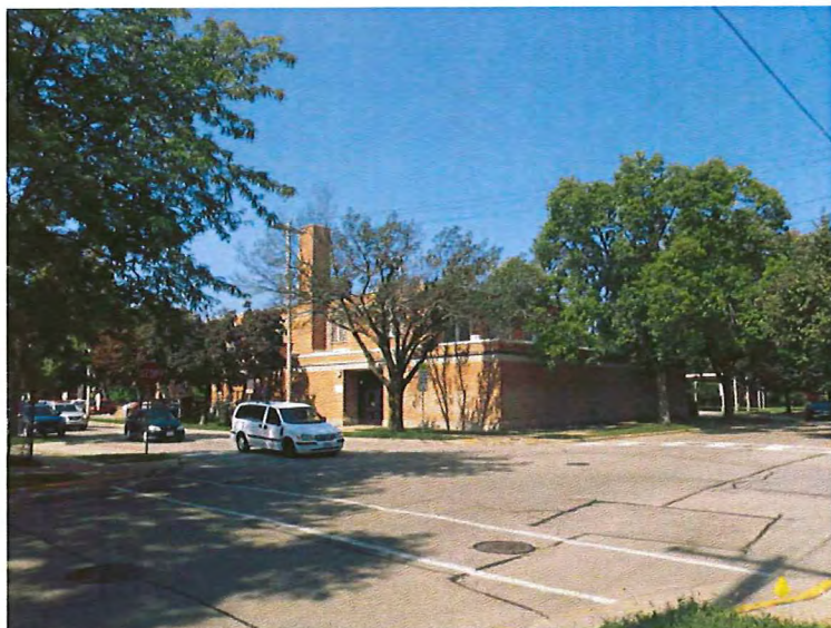
VIEW FROM MIFFLIN AND INGERSOLL LOOKING WEST
