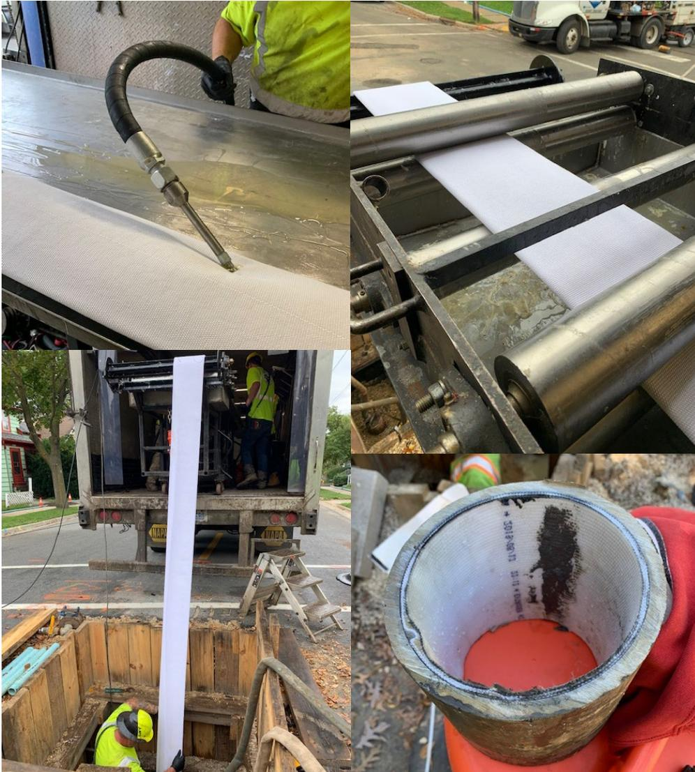
1. Woven fabric tubing, saturated with a liquid epoxy resin is pulled through the inside of the deteriorated water main between two small excavations at each end of the pipe segment.
