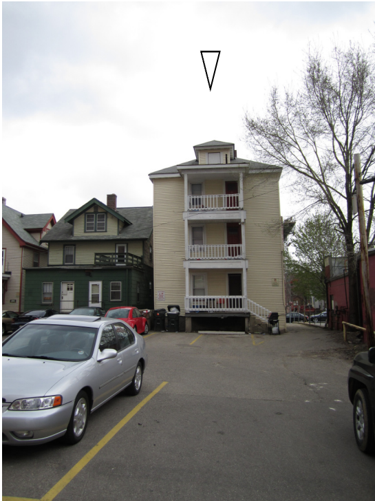
444 Johnson— rear yard elevation
