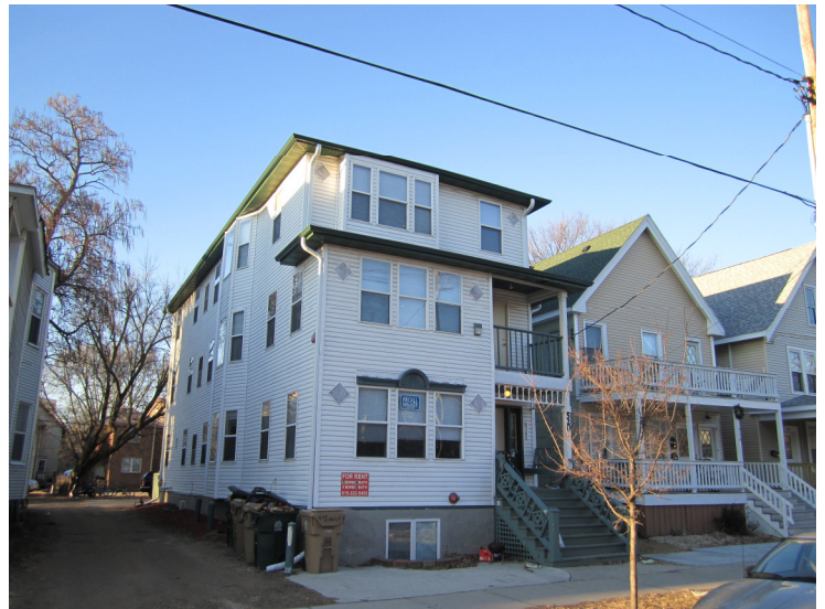
520 W Mifflin apartment building
