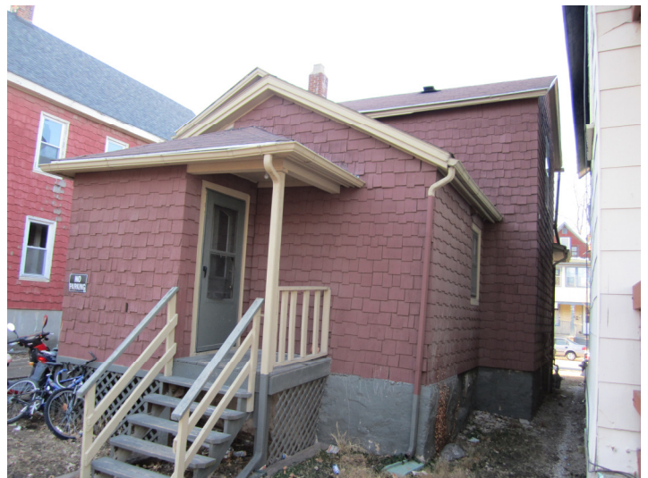
531 Mifflin existing building— from southeast
