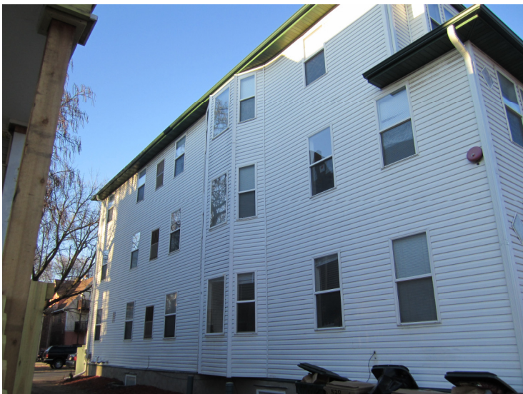
520 W Mifflin 3 story building
