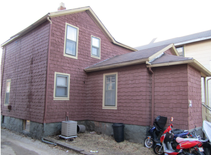
531 Mifflin existing building— from south
