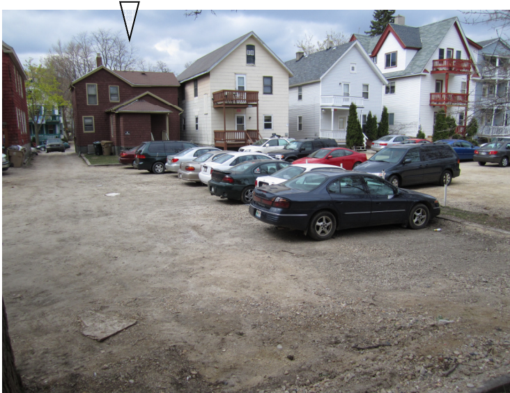
531 Mifflin existing building– rear yard and context
