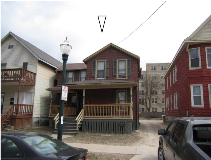
531 Mifflin existing building— street condition
