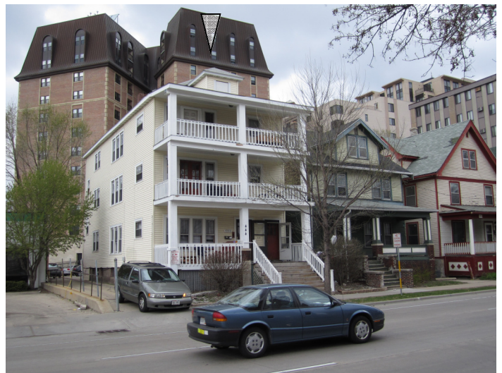
444 Johnson house— street elevation
