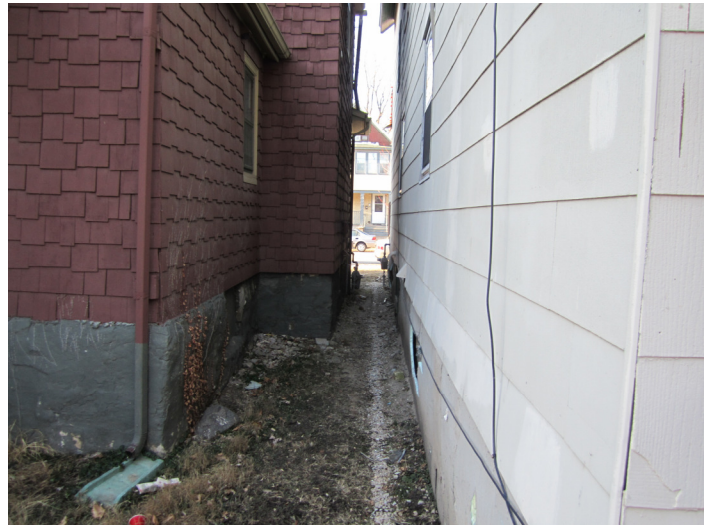
531 Mifflin existing building— northeast condition
