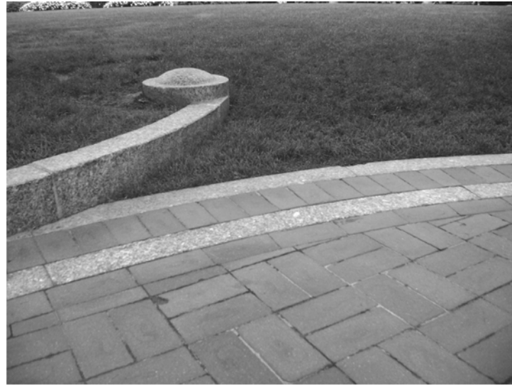
4 Lawn with Raised and Flush Curb and Unit Pavers with Contrasting Paver Trim Details SCALE: N.T.S.
