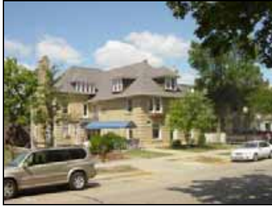
10 Langdon Morgan House Multi-Family Residential Stories – 2 to 4 Est. Elevation 99.0 Feet
