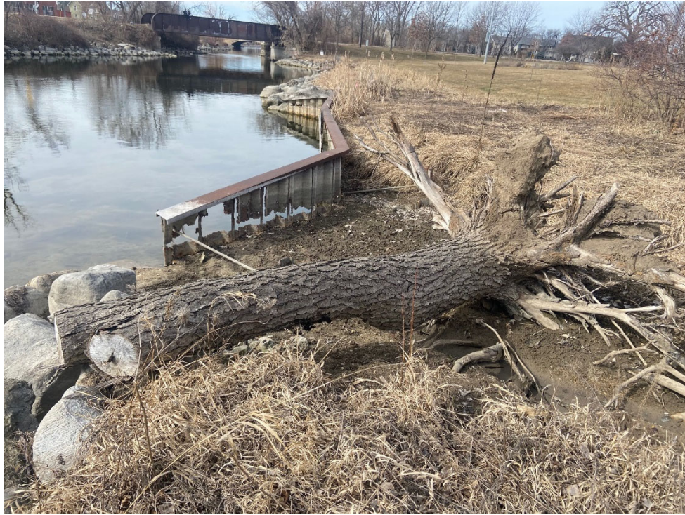
Photo 1: Existing South Seawall
