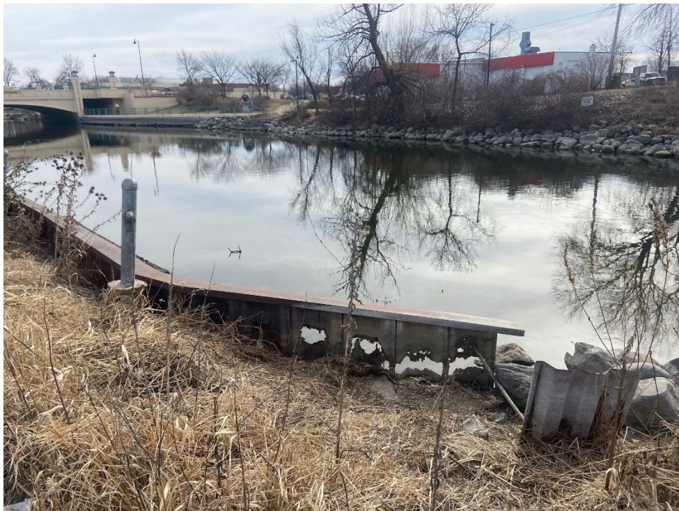
Photo 2: Existing North Seawall
