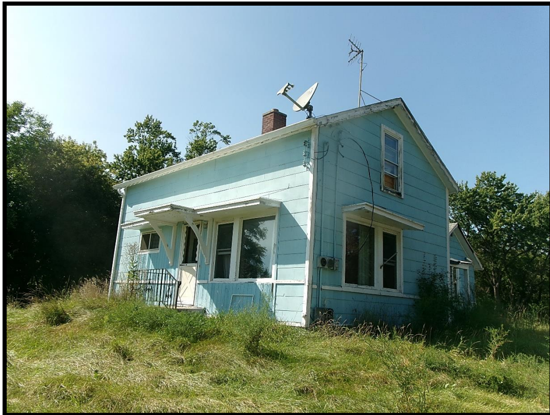
HOUSE - TO BE DEMOLISHED
