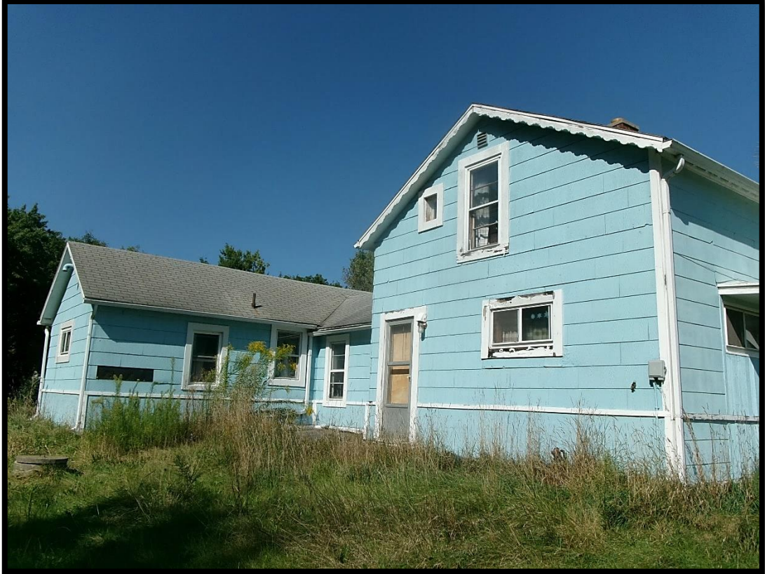
HOUSE - TO BE DEMOLISHED
