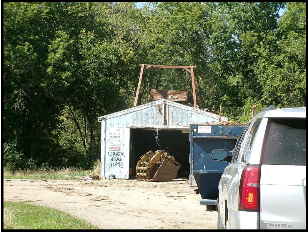
GARAGE - TO BE DEMOLISHED
