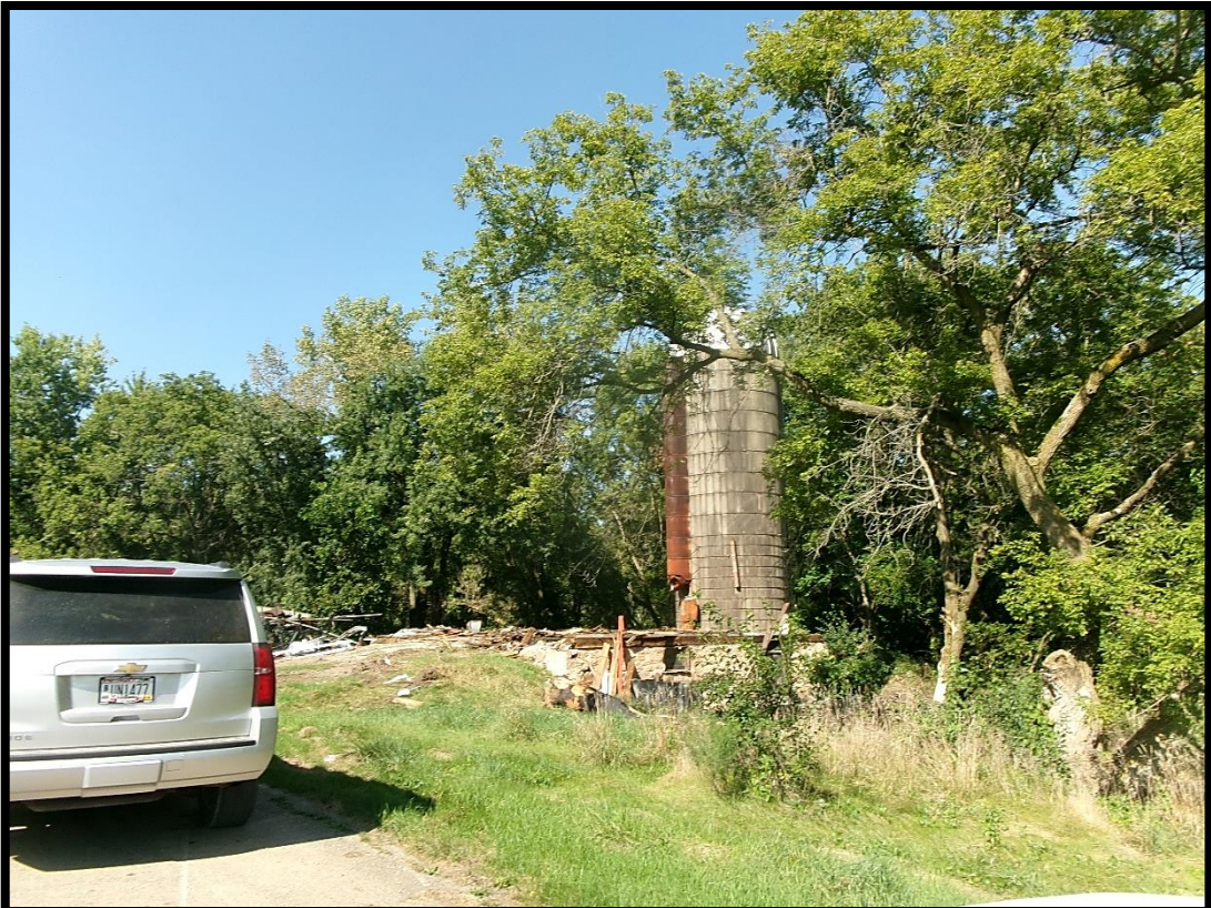
BARN FOUNDATION & SILO
