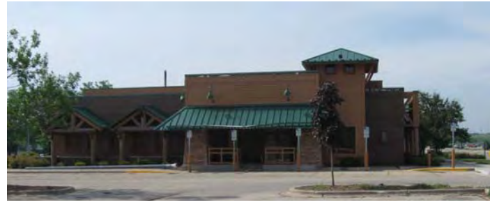
Existing Smokey Bones (to be demolished)
