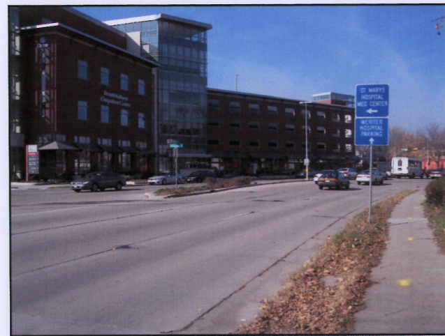
SOUTH CORNER OF LOT LOOKING NORTHWEST
