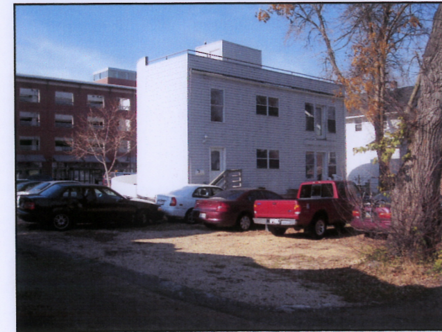
CENTER OF ALLEY LOOKING NORTHWEST
