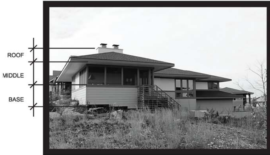
* Horizontality of Prairie Style to Conform with the Natural Contour of the Environment. Native prairie grass landscaping.
