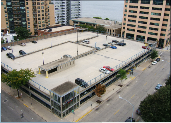
Government East Parking Garage
