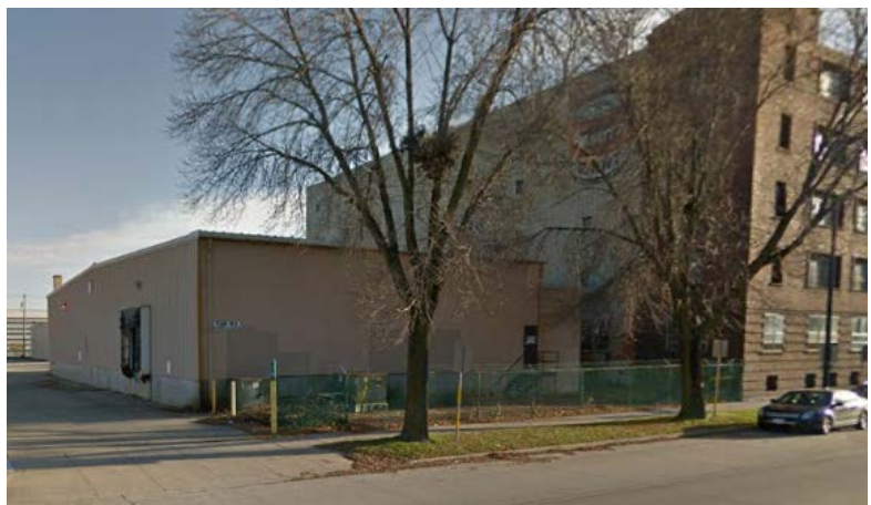
905 E Washington (1 story metal building), Google street view image
