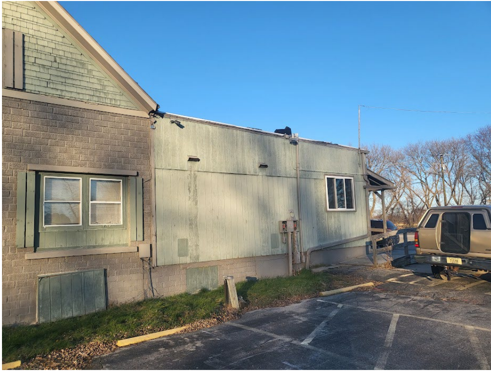
Photo 1. Southern side of building
