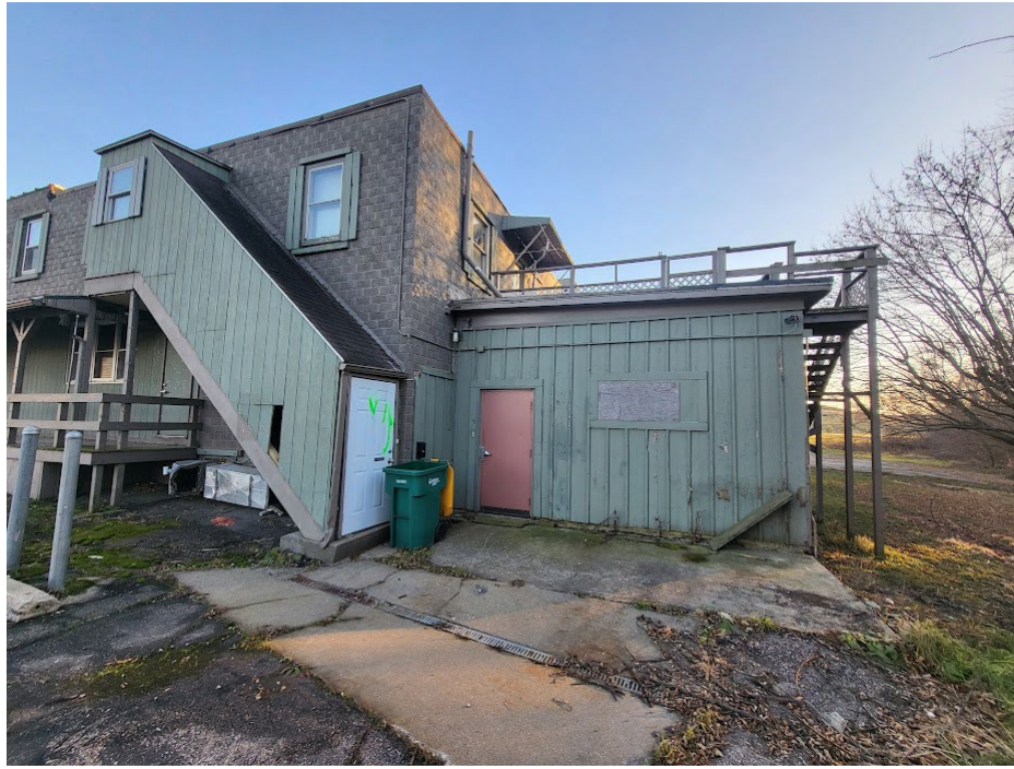
Photo 5. North stairs and basement entrance
