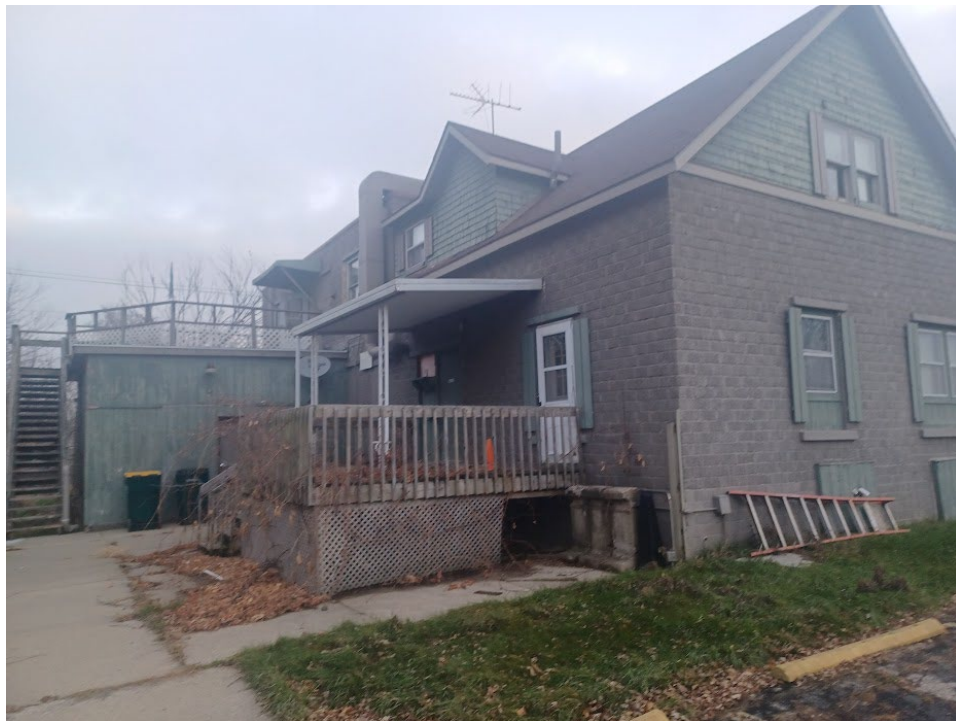
Photo 2. Western porch and stairs of building
