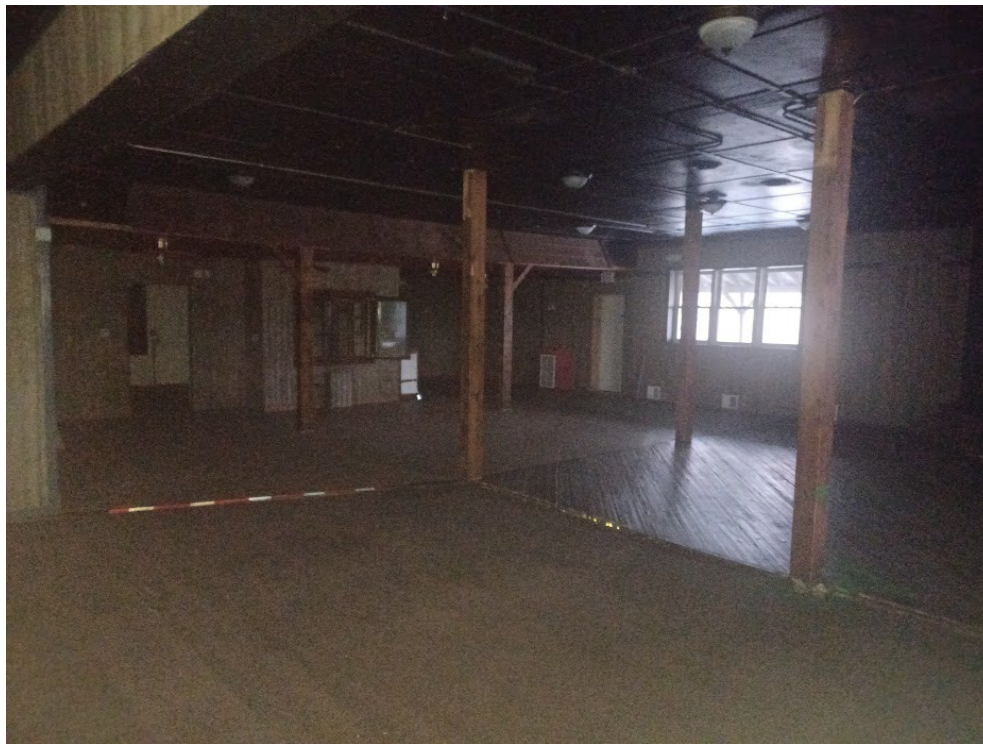
Photo 6. Main room on first floor, northern facing window
