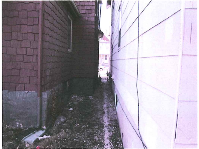
531 Mifflin existing building— northeast condition
