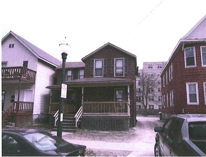
531 Mifflin existing building— street condition
