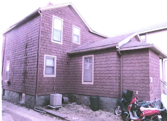
531 Mifflin existing building— from south
