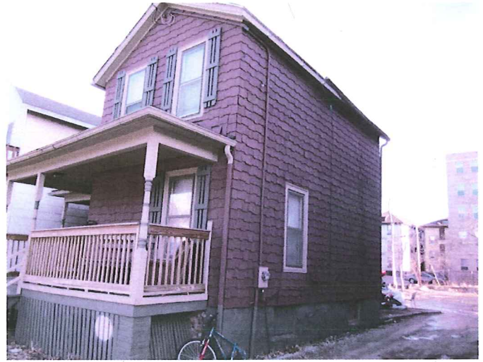
531 Mifflin existing building— from west
