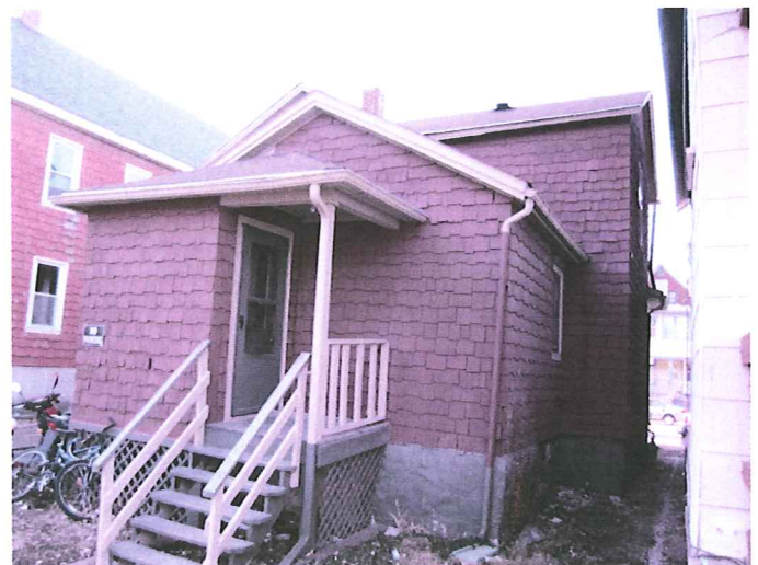
531 Mifflin existing building— from southeast
