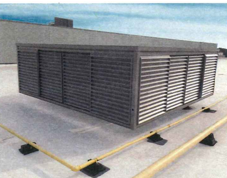
IMAGE ABOVE SERVES AS A SIMILAR EXAMPLE OF THE INTENDED ROOFTOP UNIT SCREENING SYSTEM
