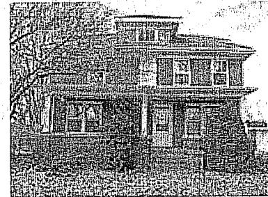
These homes, located at 3270 and 3276 Maple Grove Rd, are the future site of a new development.
