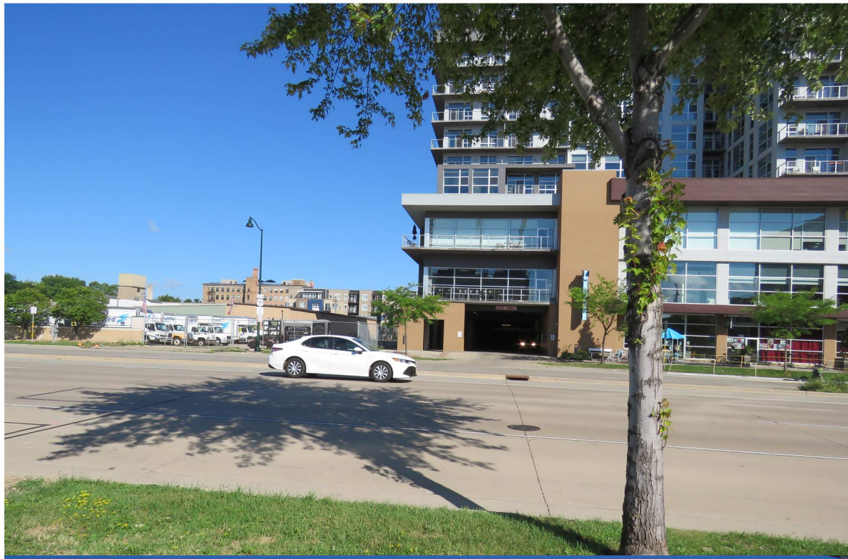
NE CONTEXT TO SITE ON E. WASHINGTON AVE
