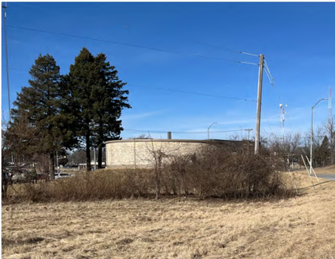
Site Photo – east of existing reservoir.
