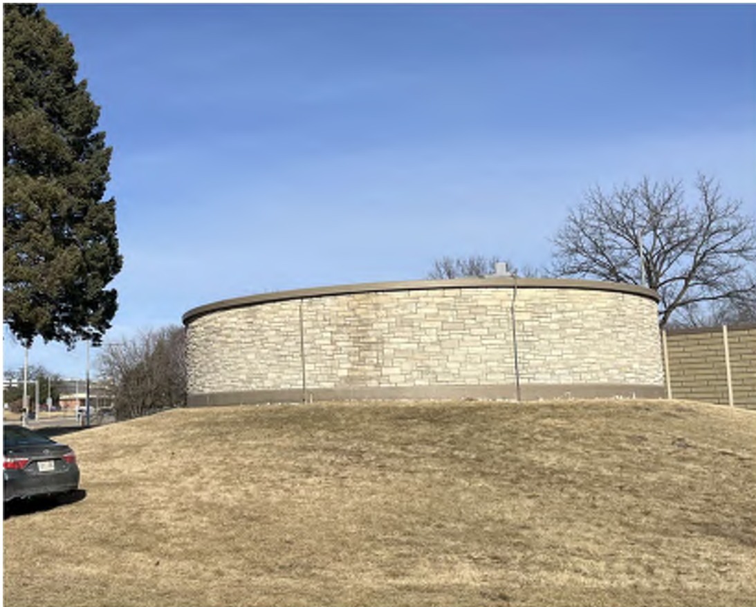
Existing Reservoir to be removed and replaced.
