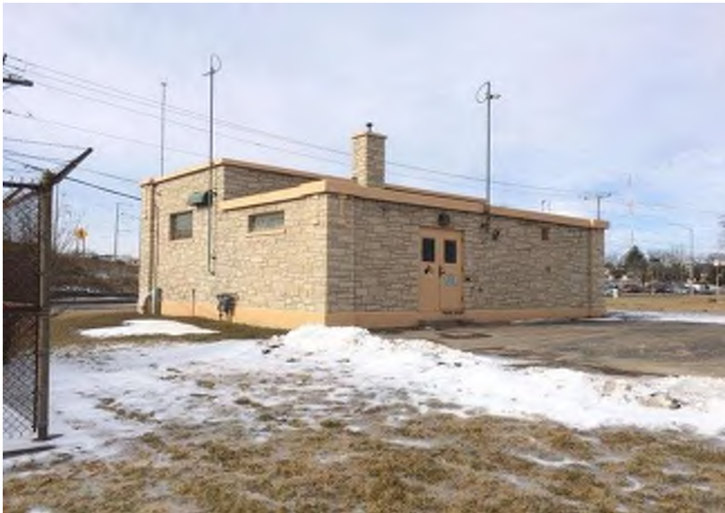
The rear of the existing Wellhouse.
