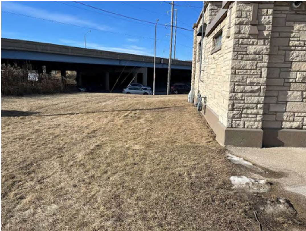
The south side of the existing Wellhouse.
