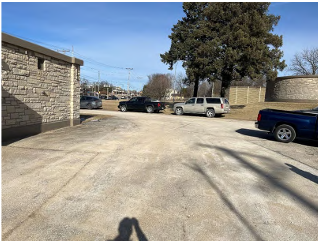
East side of existing Wellhouse.
