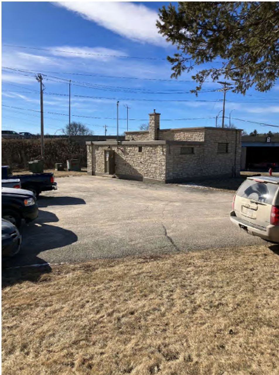
North east side of Existing Well house.
