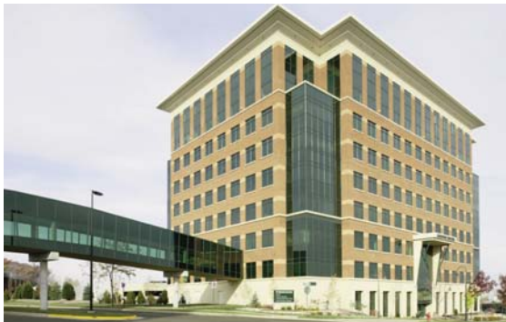
Greenway Office Building
