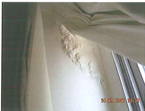
Existing damage at interior jambs due to water migration through window frames
