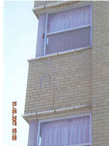
Example of brick crack repairs using sealants, now hardened over time
