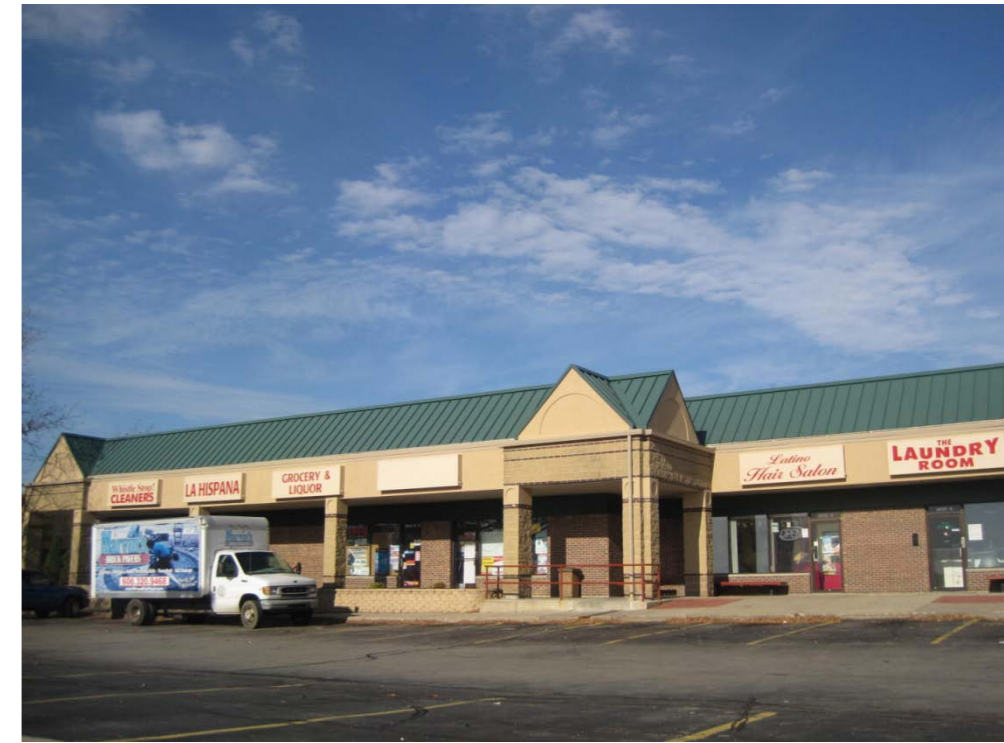
Shopping center to the north of the property.
