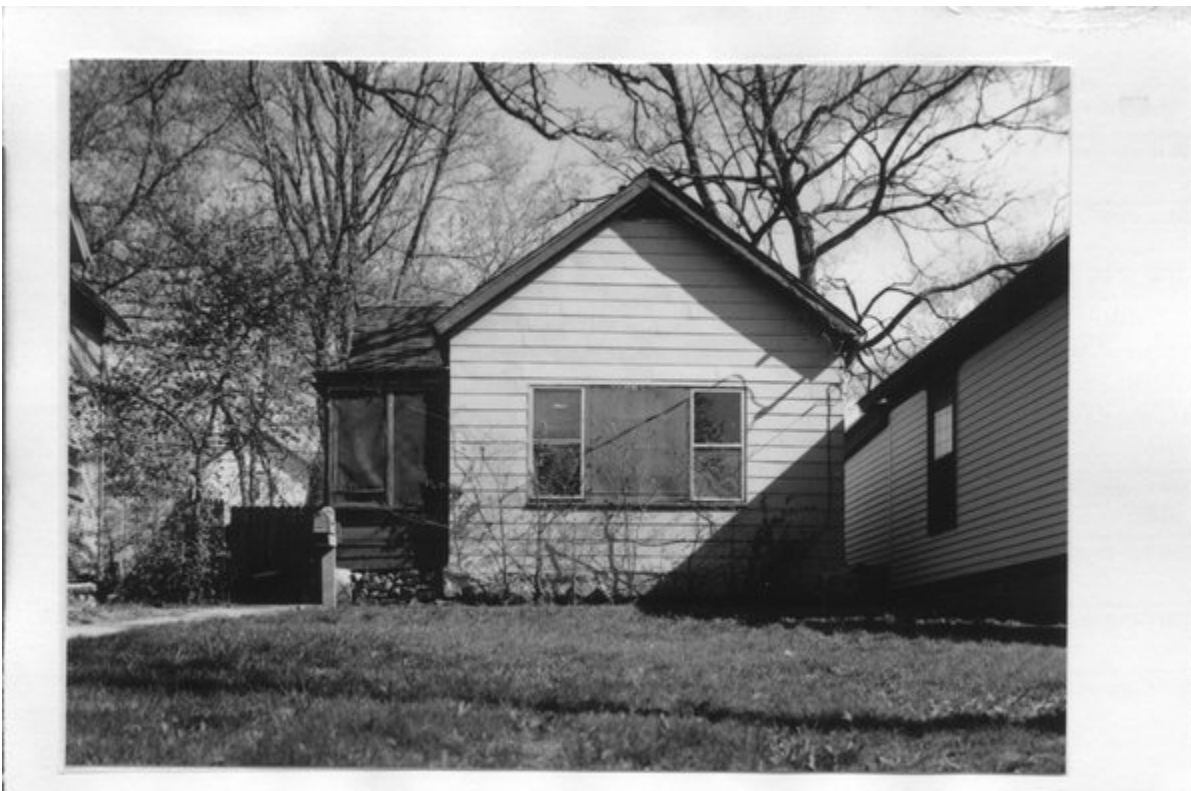
929 Williamson St. Appears to be some time before Asbestos Siding was installed in 1966. 48
