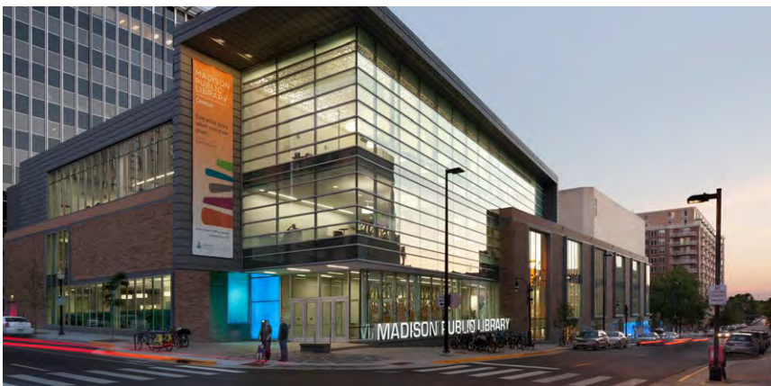
LEED Silver certified Madison Public Library Central Library An American Public Works Association National Project of the Year
