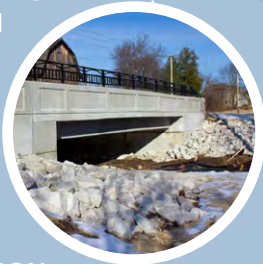
MADISON STREET BRIDGE REPLACEMENT
