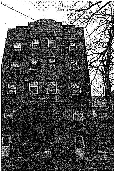
145 Iota Court – proposed for demolition
