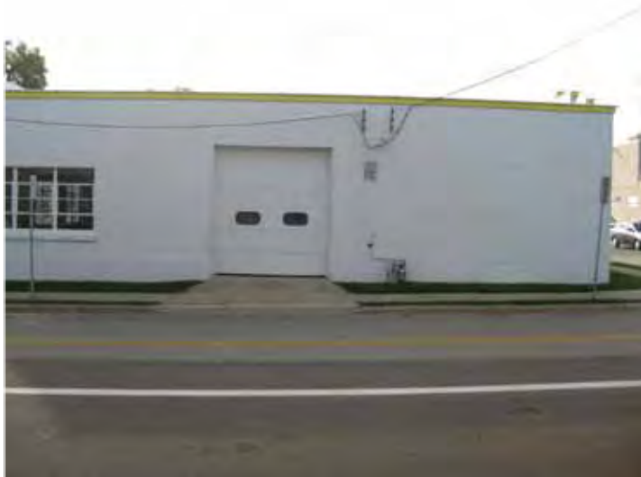
VIEW FROM PARR STREET LOOKING SOUTH
