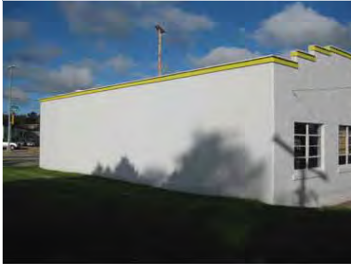
VIEW FROM 967 SOUTH PARK STREET LOOKING NORTHWEST
