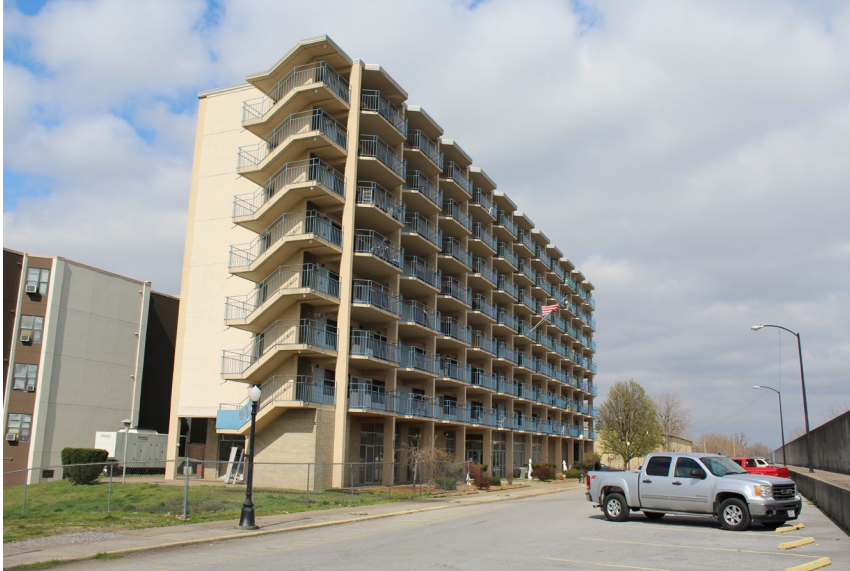
Figure 30: The U.S. Department of Housing and Urban Development (HUD) proposed demolishing the Connell F. Smith Sr. Building in Cairo, Illinois, the area's fifth public housing complex to close. Sixty residents will be displaced in a community already experiencing a severe affordable housing shortage. Landmarks Illinois has joined with residents, housing advocates and other government agencies calling for HUD to create new affordable housing in Cairo. Photo by Don Patton, Cairo Historical Preservation Project.
