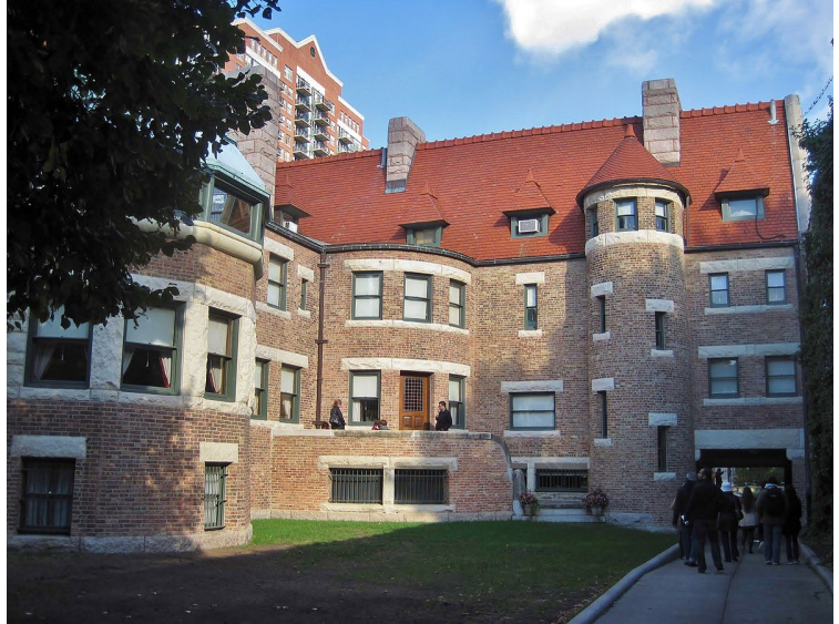
Figure 38: The Glessner House in Chicago , Illinois, had a geothermal system installed under its interior courtyard to reduce energy costs with no visual impact on the National Historic Landmark home. Photo by Teemu008 from Palatine, Illinois, October 19, 2013, CC BY-SA 2.0. Photo unchanged.
