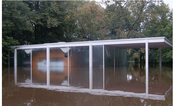
Figure 41: Water levels are rising beyond the U.S. coastlines. Extreme weather events, coupled with development, has led to rapid river rise in many parts of the world. The Edith Farnsworth House in Plano, Illinois, built right next to the Fox River, was designed by Mies van der Rohe to withstand minor floods, but not frequent, major flooding. The National Trust for Historic Preservation, the home's owner, and Landmarks Illinois, preservation easement holder, have been exploring flood remediation options. Photo by Landmarks Illinois.
