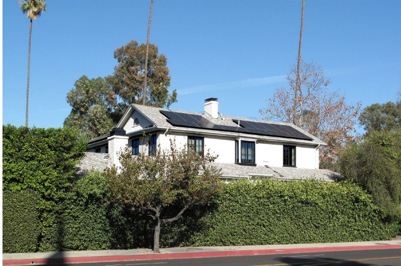
Figure 37: Solar panels on the roof of a Los Angeles home in the Hancock Park neighborhood. Much of Hancock Park is in a municipal Historic Preservation Overlay District. California State Law exempts solar installations from requiring municipal clearance, including in historic districts. Photo by Downtowngal, January 21, 2021, CC BY-SA 4.0. Photo unchanged.
