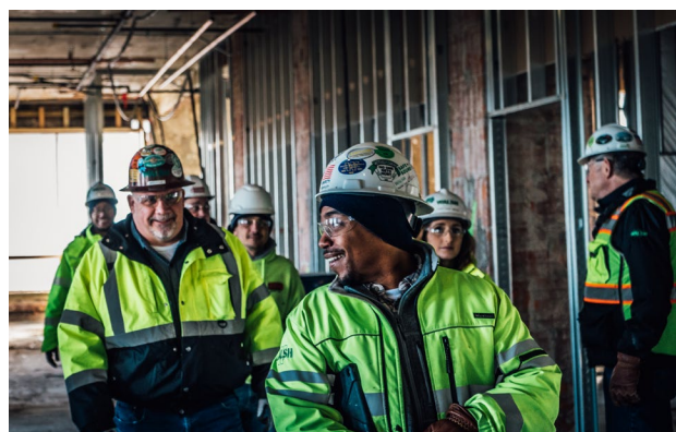
Figure 50: Walsh Construction sponsored a Pre-Apprentice Program where candidates gained experience participating in the historic Cook County Hospital renovation . Photo_by_Torque, provided by Walsh Construction.
