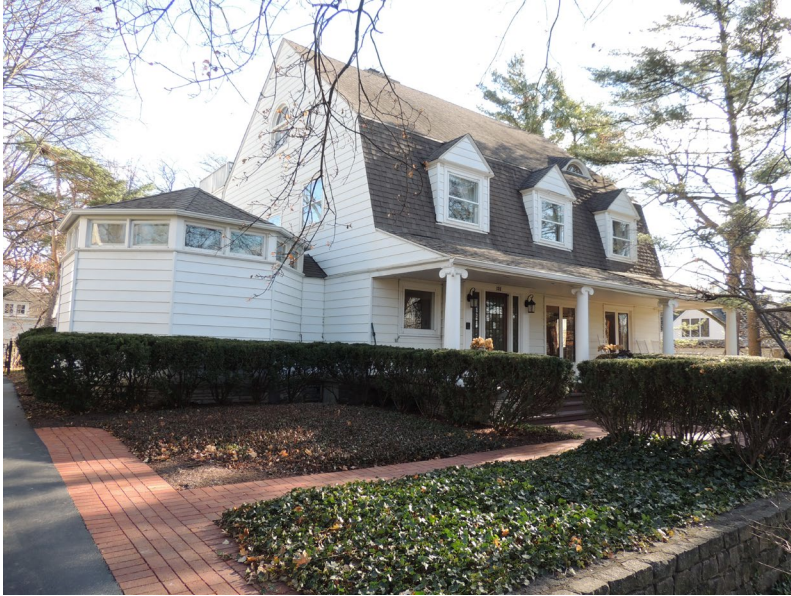
Figure 9: The Frank Lloyd Wright-designed Frederick Bagley House in Hinsdale, Illinois was saved at the 11th hour after fears it would be a teardown. The State Historic Preservation Office suggested that the home can't be nominated to the National Register for architectural significance until the replacement aluminum siding is removed that covers the original wood shakes underneath. Photo courtesy of Jean Follett.
