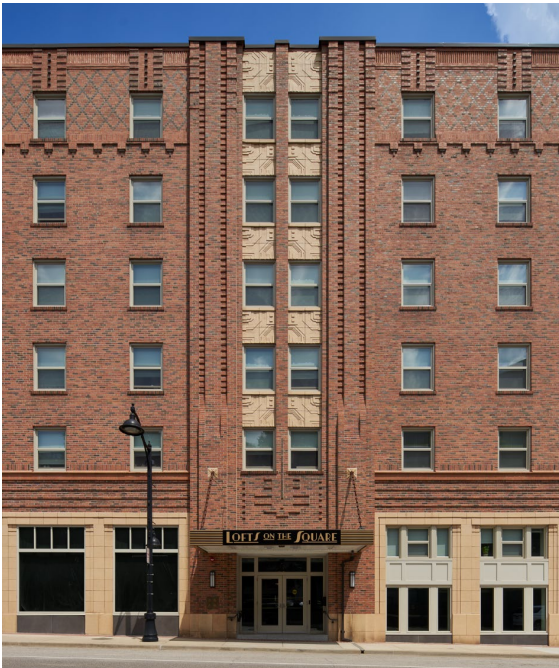
Figure 27: Working with the local government and advocates, Landmarks Illinois (LI) helped find a developer to reuse the vacant, former Hotel Belleville in Belleville, Illinois. With AIA Illinois, LI helped pass the state's 2018 rehabilitation tax credit making additional financing available. Renamed Lofts on the Square, the building now provides 47 affordable senior housing units. Photo by Andrew Bruah Photographer and used with permission.
