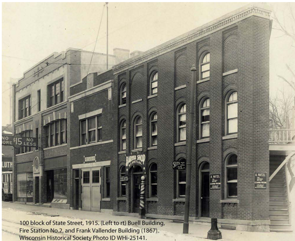
Vallender Building (rt), 127-129 State Street, Madison, WI, circa 1905. Dorothy Park Collection, Wisconsin Historical Society Photo ID WHI-23434.
