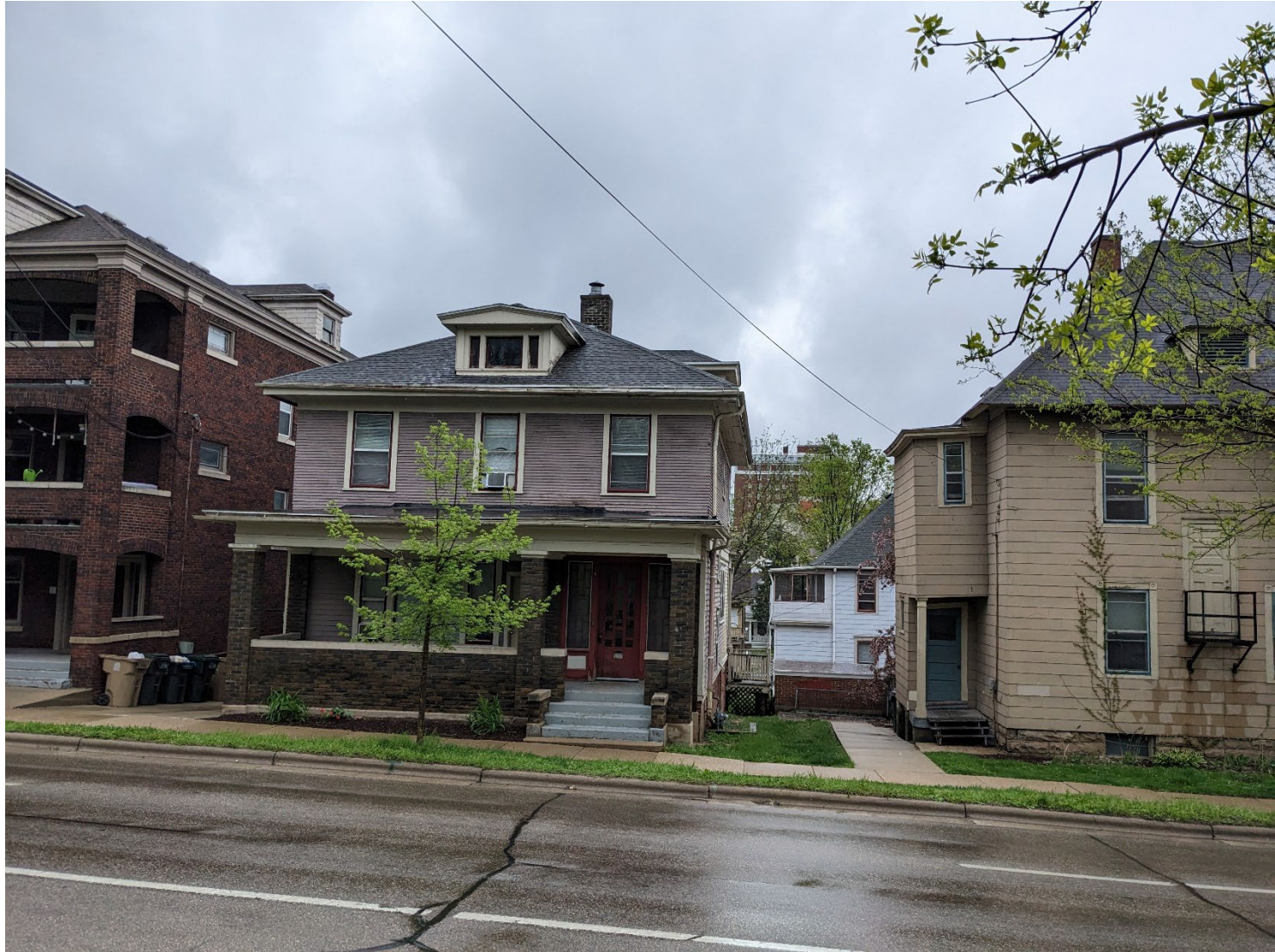
Front North Elevation – View from Gorham St
