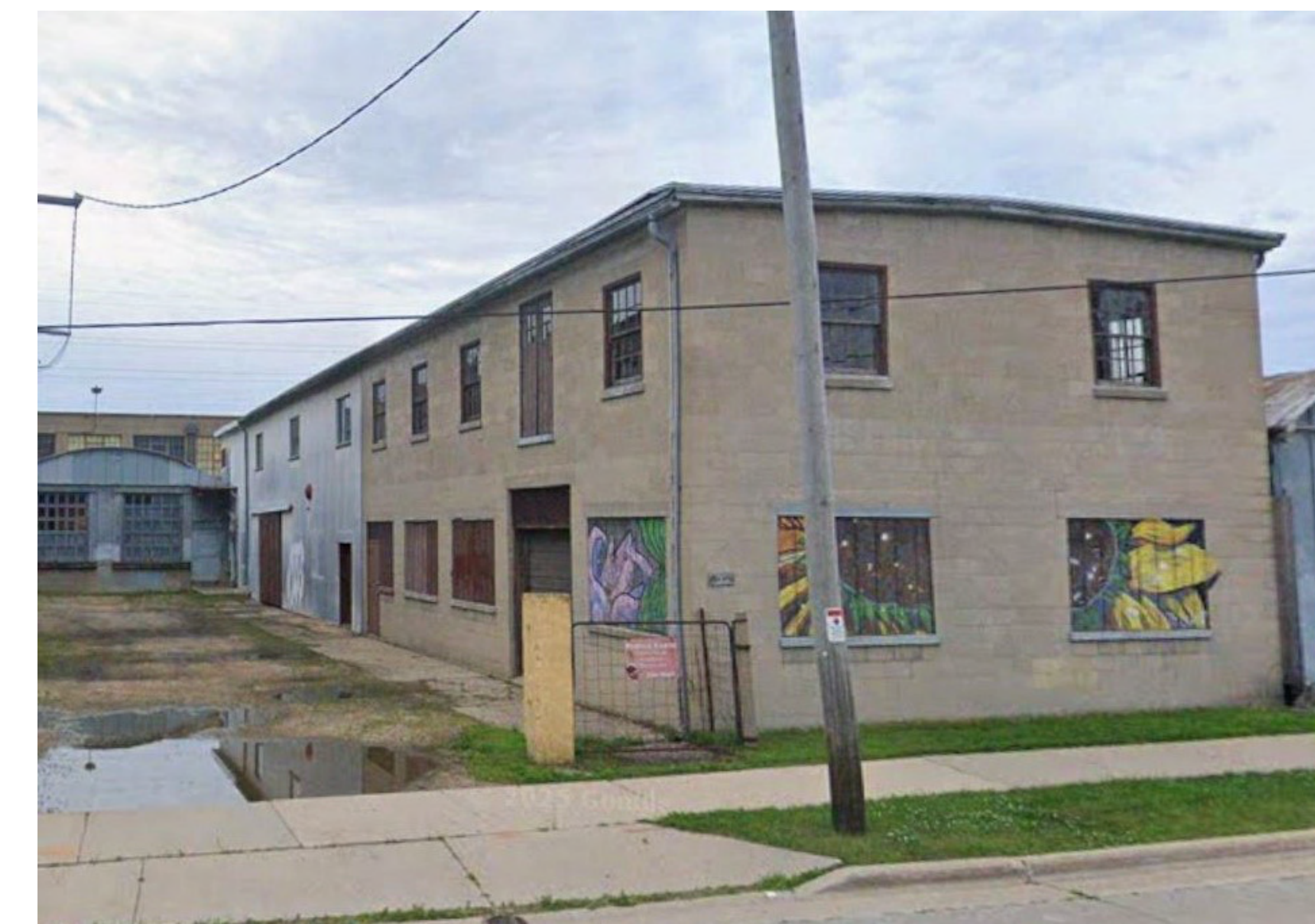
1902-2010 PENNSYLVANIA (WAREHOUSE BLDG)
