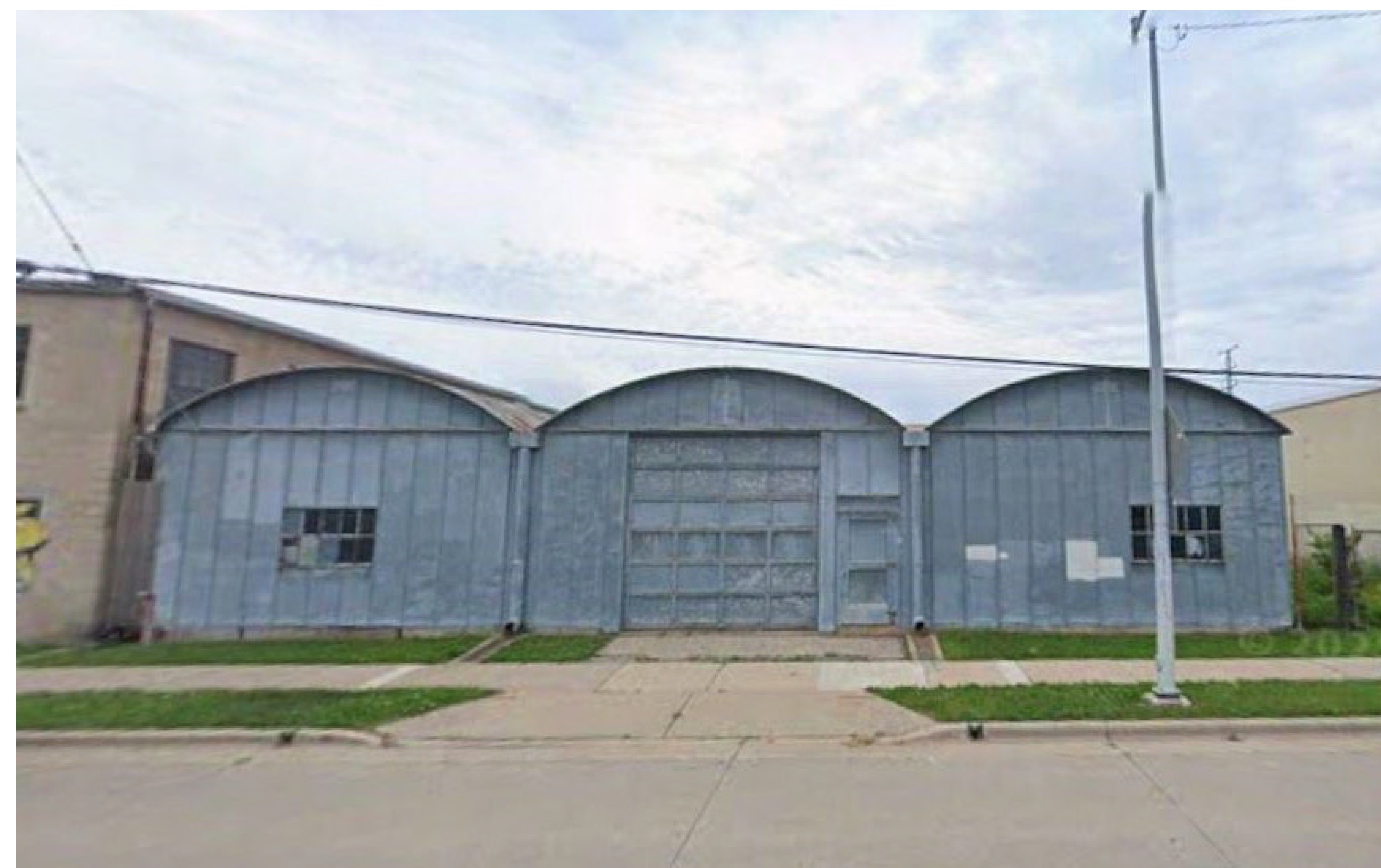
1902-2010 PENNSYLVANIA (WAREHOUSE BLDG)
