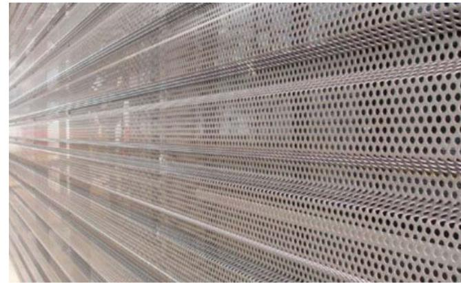
3' TALL PERFORATED, CORRUGATED AC CONDENSER SCREENING PANEL, GALVALUME
