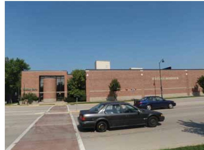
VIEW FROM EAST WASHINGTON OF EXISTING MADISON DAIRY
