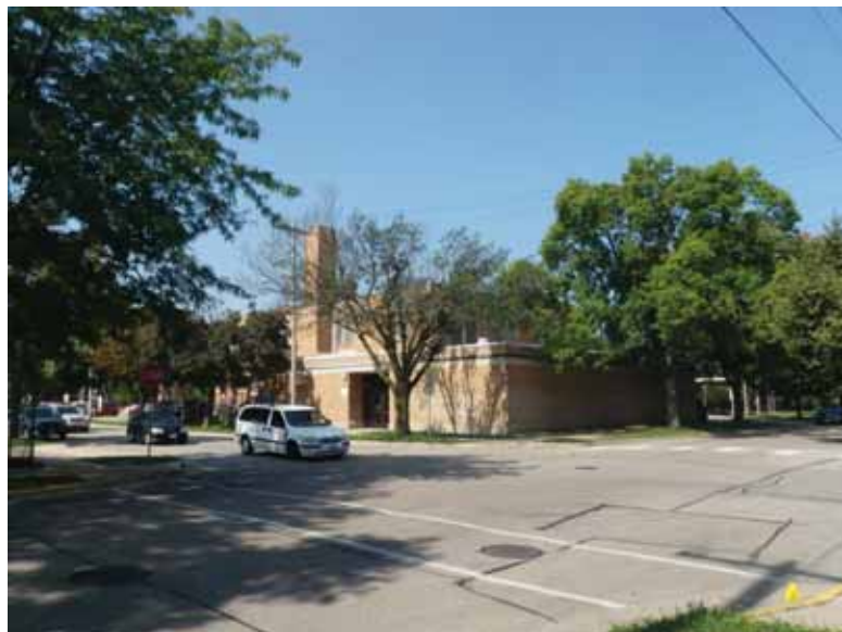
VIEW FROM MIFFLIN AND INGERSOLL LOOKING WEST
