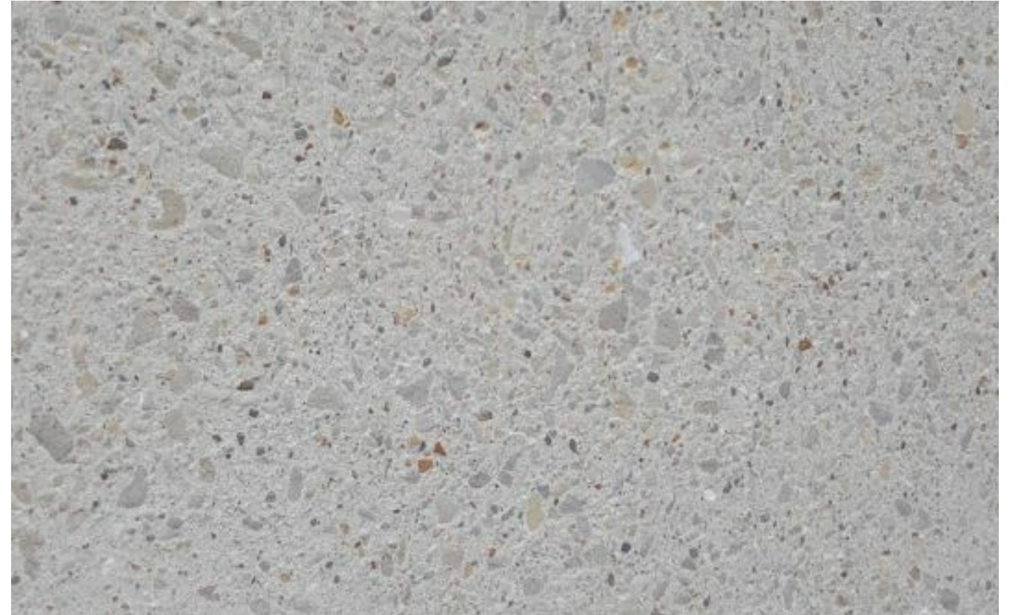
SAND BLASTED TILT-UP CONCRETE WALL
