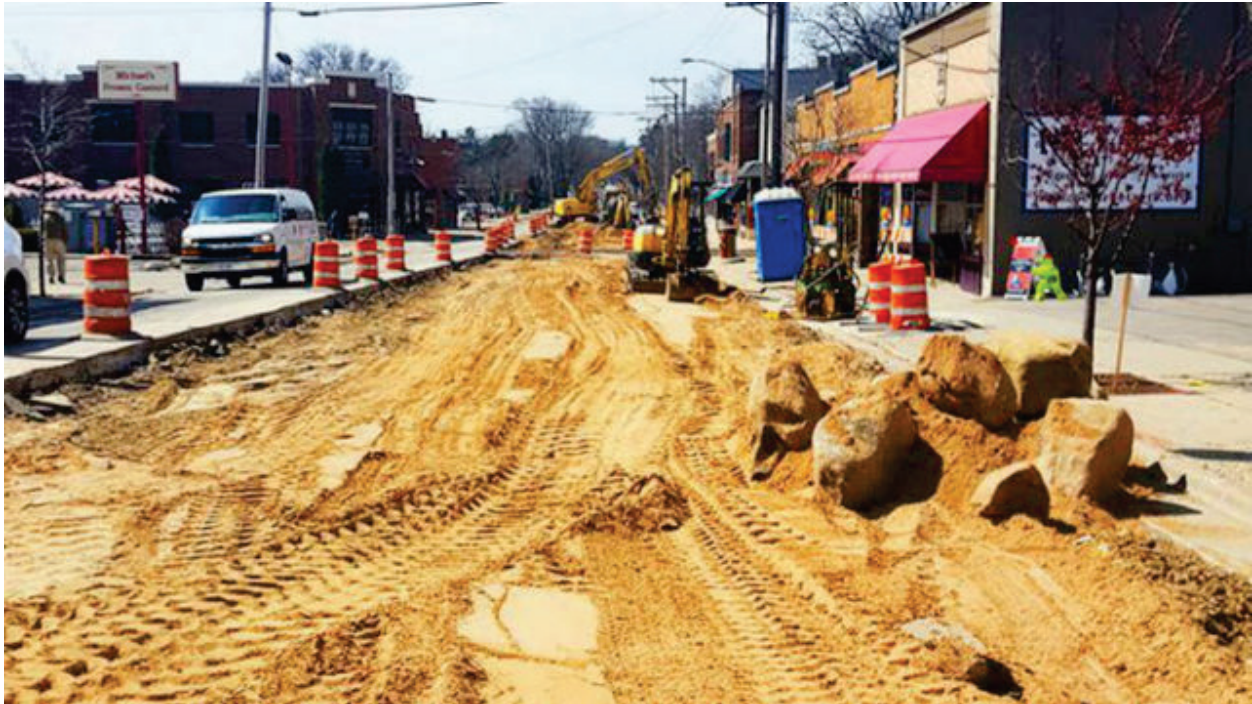
Monroe Street Construction
