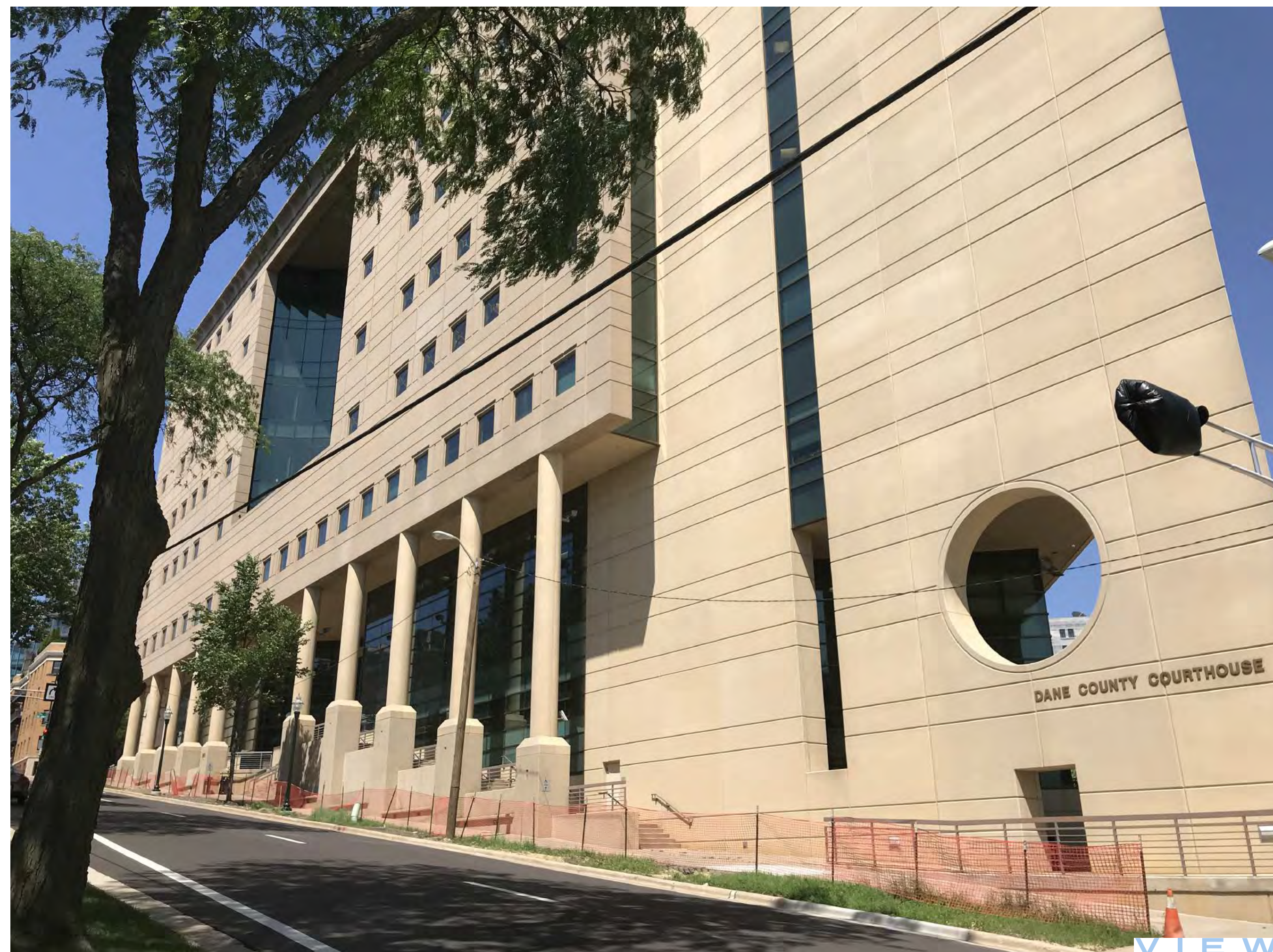
DANE COUNTY COURTHOUSE
