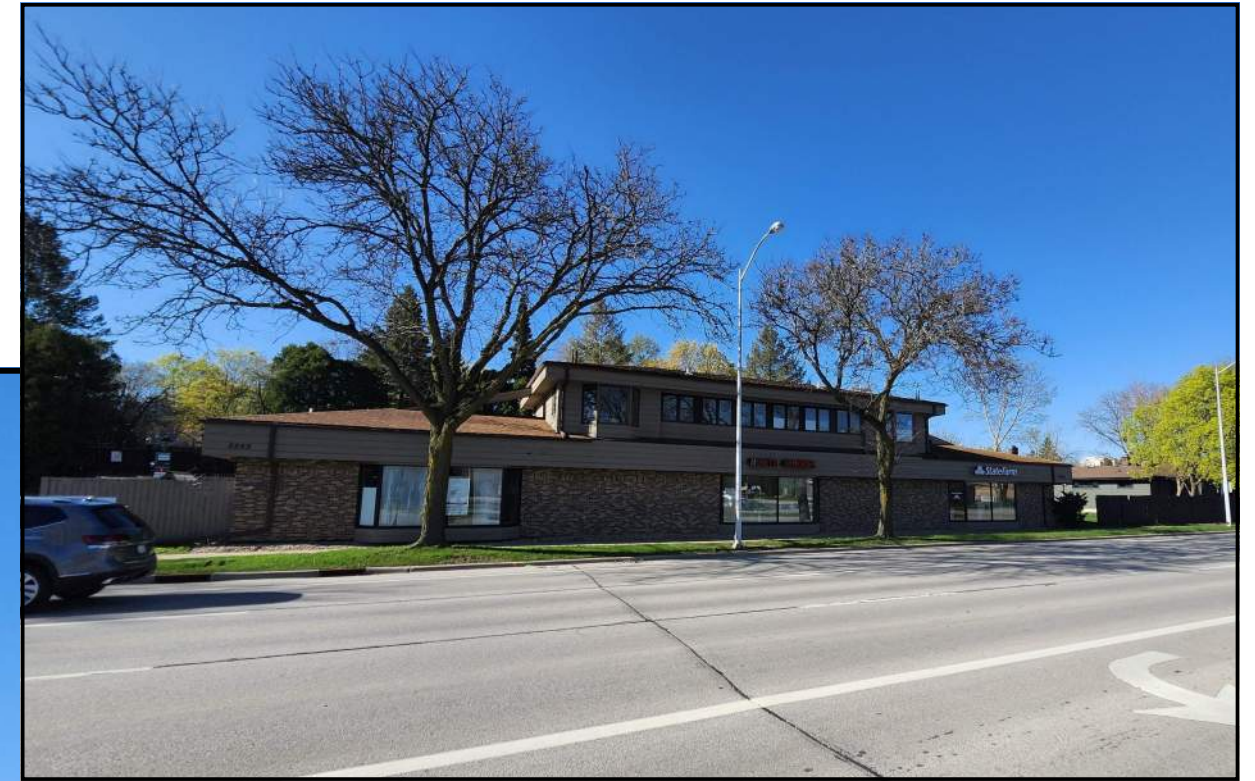
EXISTING WEST BUILDING 3553 UNIVERSITY AVENUE
