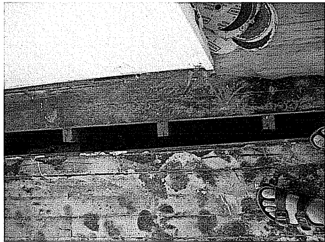
The floor joist down the center of the cabin separated by 2 inches the entire length of the structure
