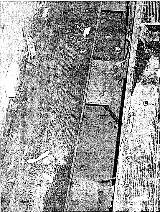
The floor joist down the center of the cabin separated by 2 inches the entire length of the structure
