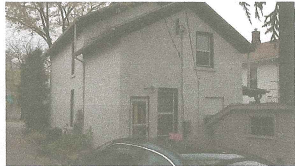
View of Rear
