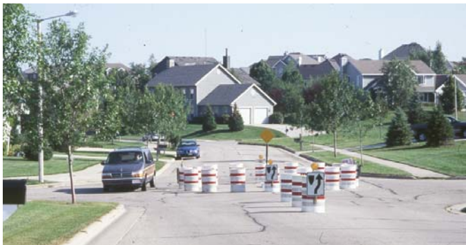
Temporary installation of a traffic circle at New Washburn way and Dandaneau Trail
