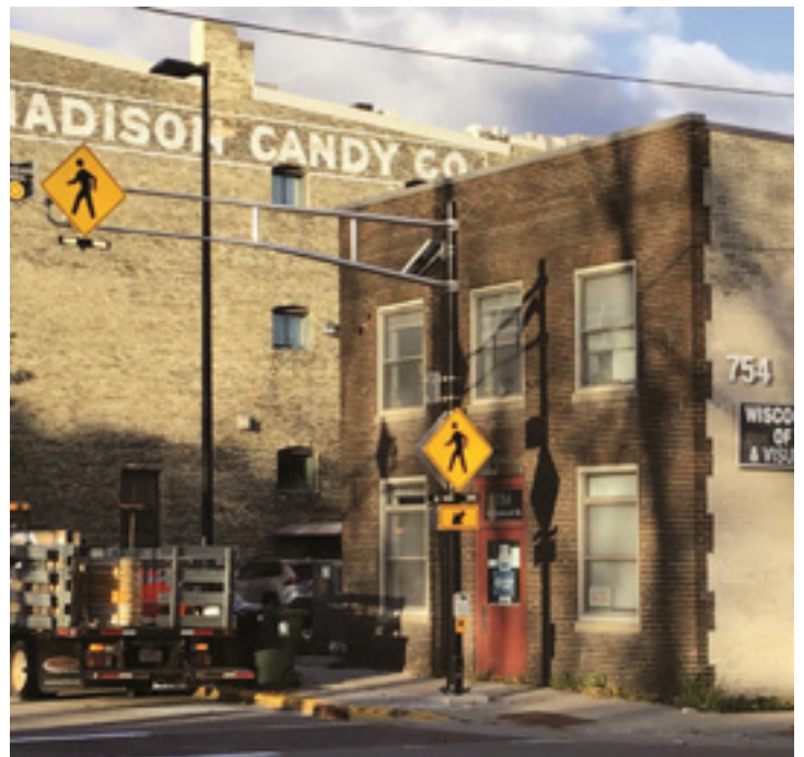
Crosswalk beacon improves pedestrian safety at the intersection of Williamson and Livingston Streets
