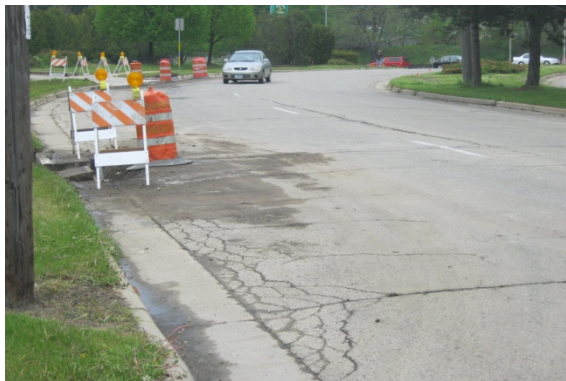
Whitney Way (under construction – not evaluated)
