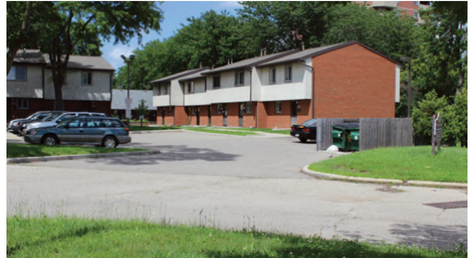
FIGURE 9 View of Parkside Apartments demonstrating a typical arrangement of housing within the Triangle neighborhood, which focuses front doors inward towards the parking lot.
