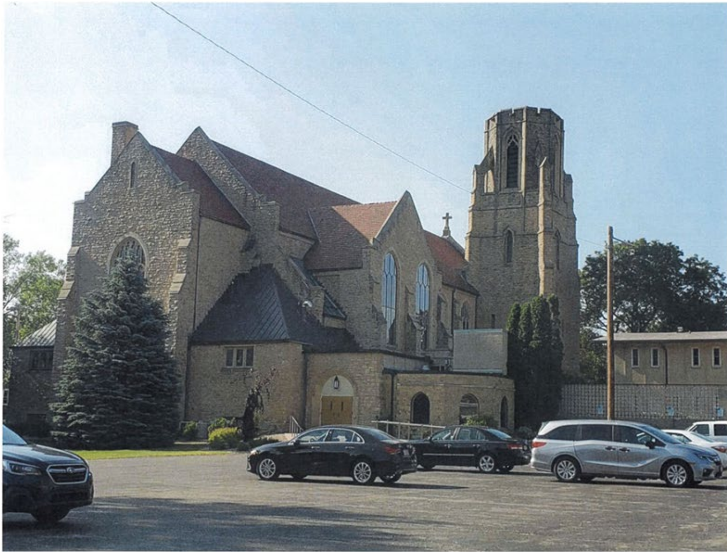
PARKING LOT ENTRANCE
