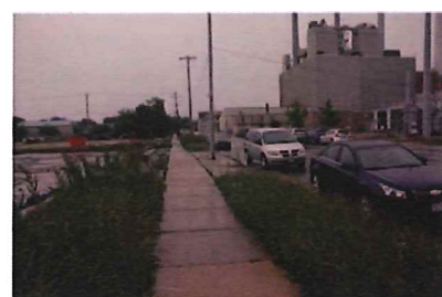
VIEW FROM E. WASHINGTON AVE LOOKING SOUTHWEST
